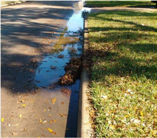
Dead leaves accumulating along the curb prevent runoff flow to storm drain
