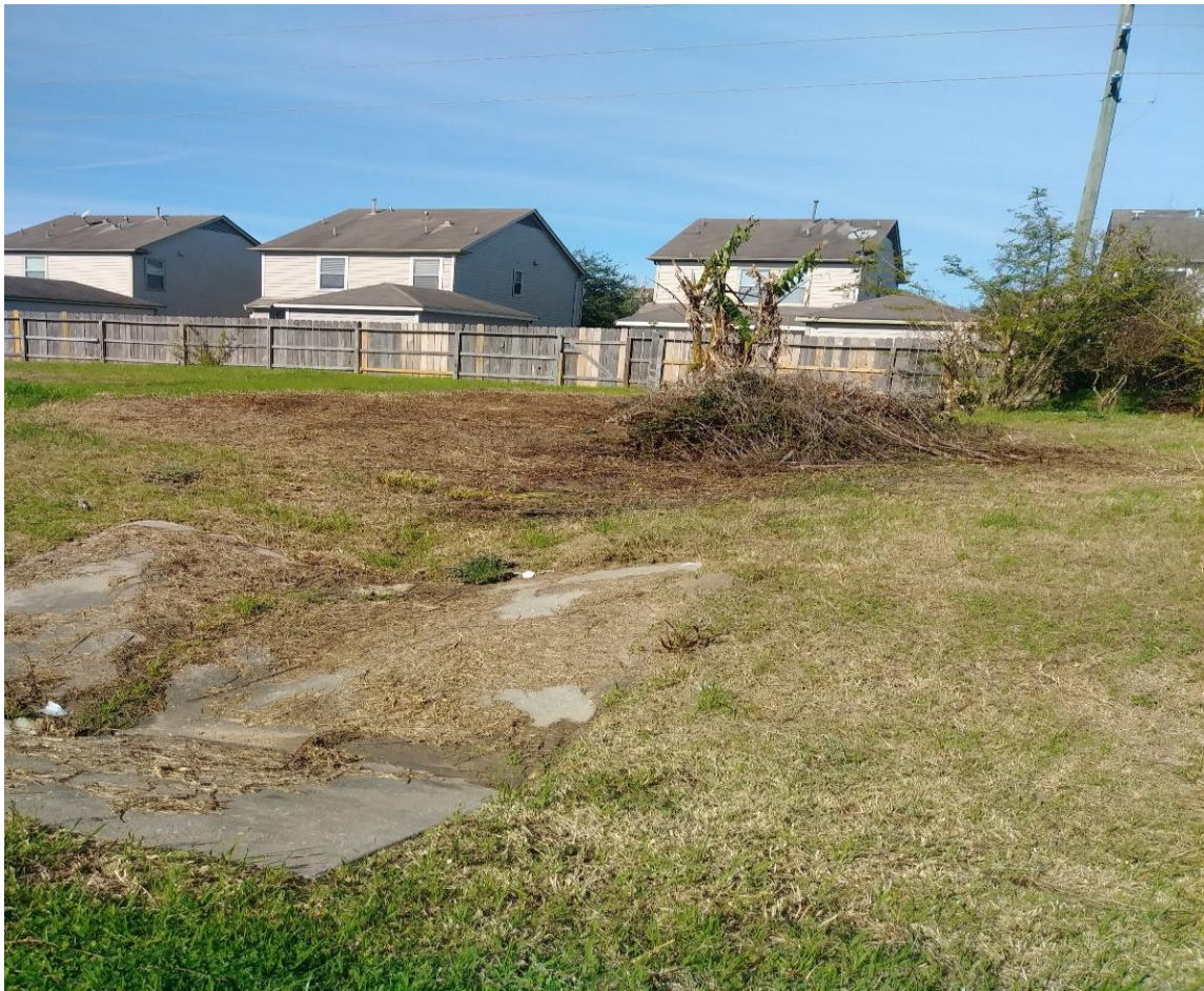
Dumped tree trimmings and other yard debris block the flow of runoff into the flood control swale and drainage channel
