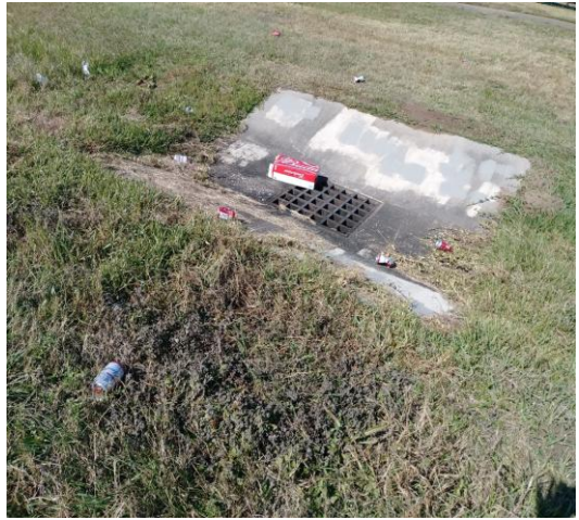
Beer cans and box tossed onto swale grating will make their way into the drain
